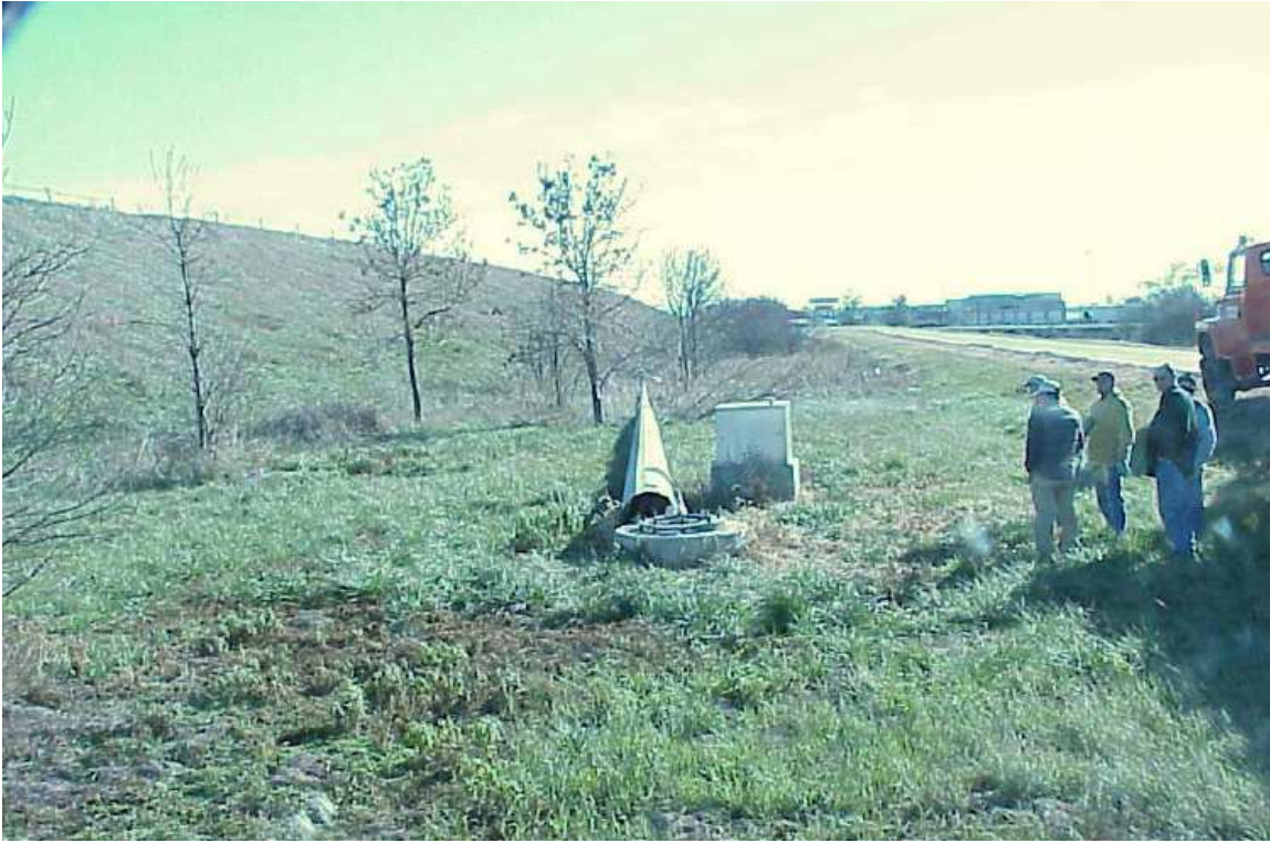
Figure 1-1. A collapsed high-mast light pole along I29 near Sioux City in 2003 [3]
